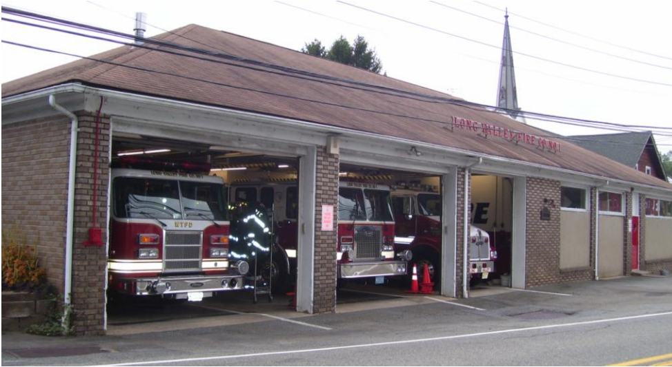
WTFD -- Long Valley Fire Company
