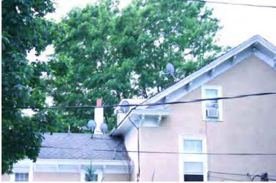
Four satellite dishes on a single building.....
