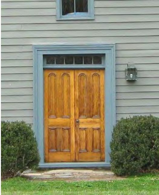
Although these doors in the Middle Valley District are most likely not original to the house, they have achieved historic significance over time.
