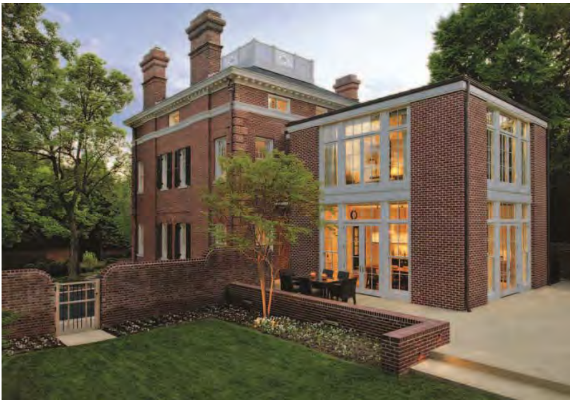
This glass and brick structure is a harmonious addition set back and connected to the rear of the Colonial Revival-style brick house. Cunningham/Quill Architects. Photos: © Maxwell MacKenzie.
