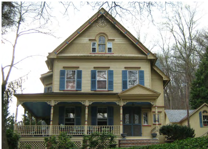
One of the more ornate houses which displays a combination of wood siding types.
