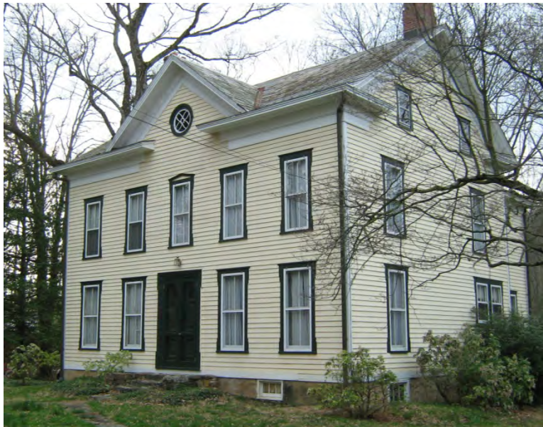
Typical cross gable in the Middle Valley Historic District.
