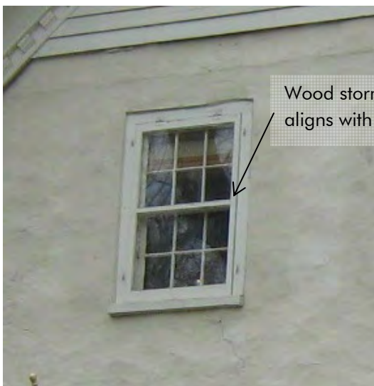
Historic sash remains behind exterior storm.
