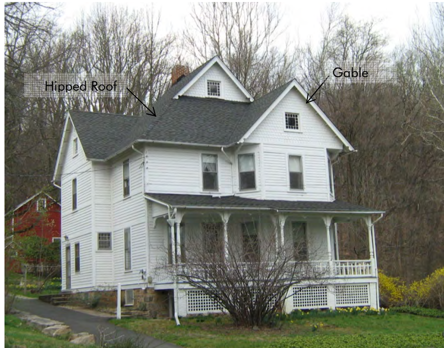
Combination hipped and gable roof forms at this simple Queen Anne along Schooley's Mountain Road.
