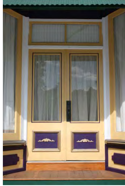
Double doors at store front in the German Valley District.
