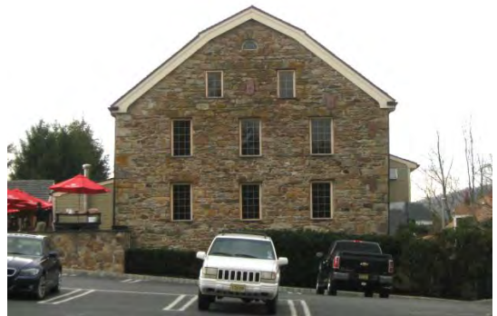
The gambrel roof of the large stone barn (now a restaurant) is one of three gambrel roofs in the districts.
