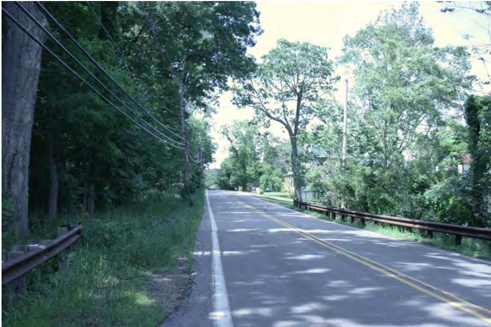
View north along Schooley's Mountain Road.
