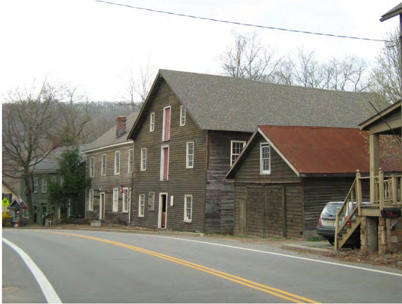
Mix of early commercial and residential buildings in the German Valley Historic District.
