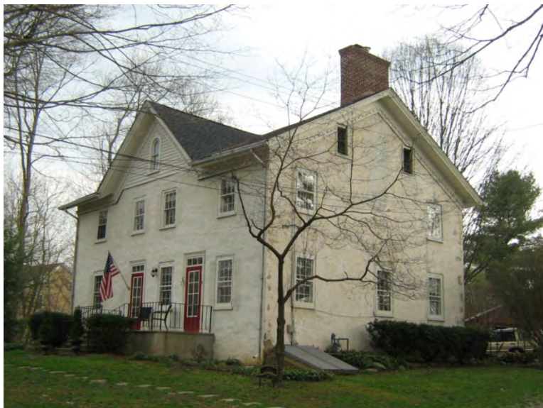
Converted cross gable.
